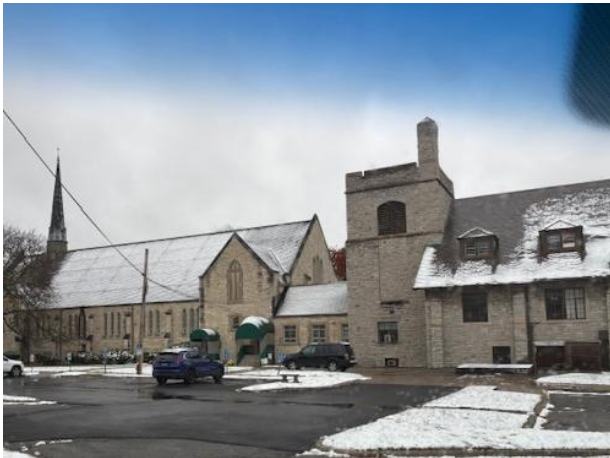
Above: Monroe Street United Methodist Church: The Bridge Ministry & Neighborhood Center
