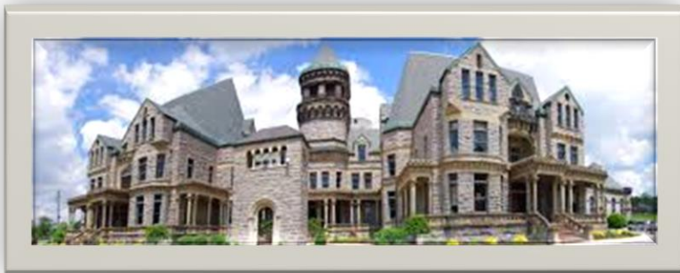
Left: Front of the Ohio State Reformatory in Mansfield, Ohio.
